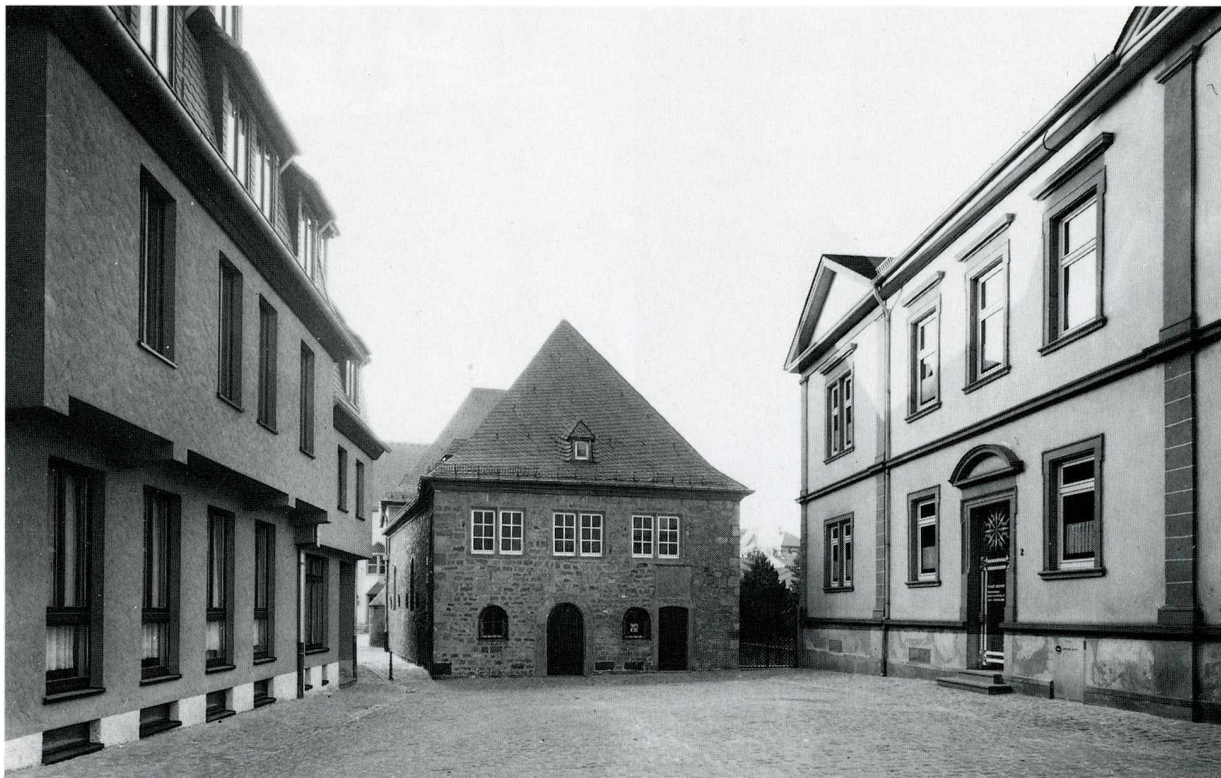
Synagogenplatz with house "to the Sun" (right), synagogue vestibule, and entrance to the courtyard
