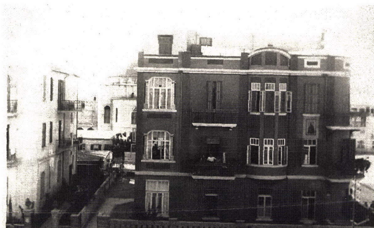
A typical apartment house in Tel-Aviv
