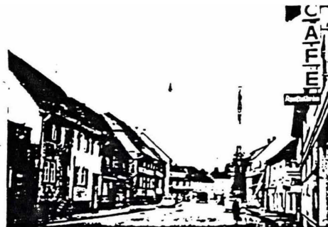
Hauptstraße - The greater portion of the buildings/houses was once owned by Jews
