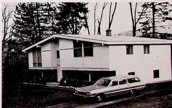
ONE OF THE NEW HOUSES
